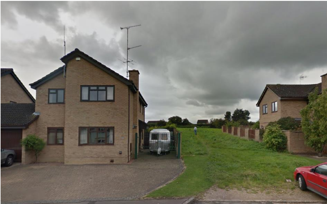
Plate 1 Entrance into the SUB09 site from The Wheatfield East
